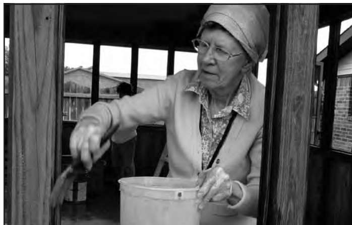
ELCA volunteer Pearl Anderson stains the spring house at the home.
